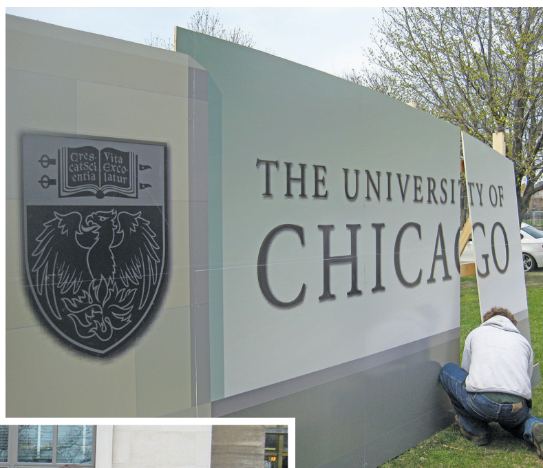
Gehshan says the stone and glass gateways for the University of Chicago were also tested in mockup form; it was especially important to confirm the appearance and scale inexpensively before the gateways were constructed. Collaboration with the fabricator greatly enhanced the effectiveness of the project. (Image courtesy of Cloud Gehshan Associates)
